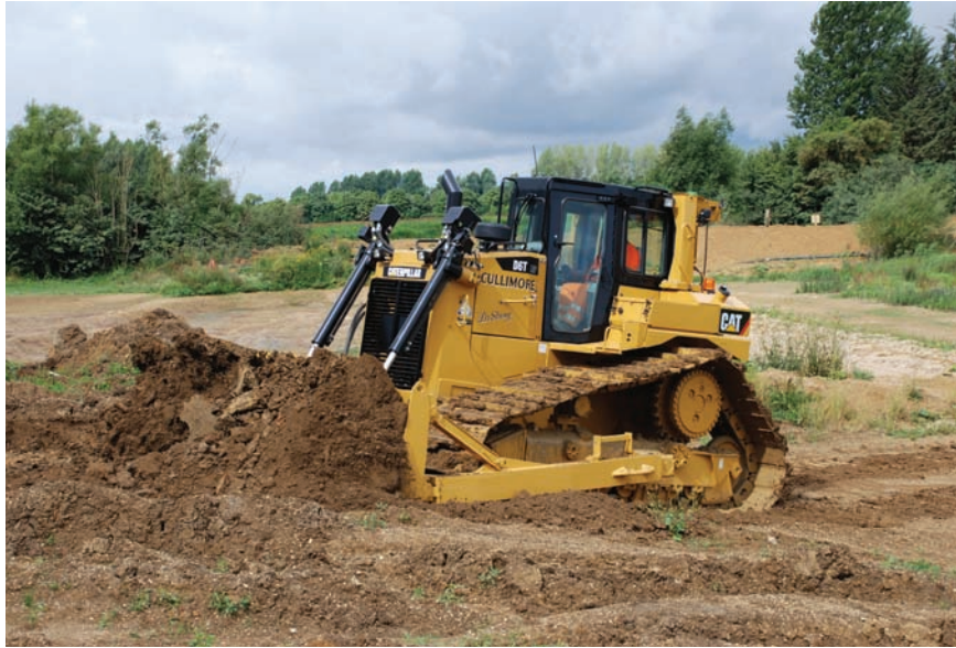
Earthmoving operations at a Cullimore site
